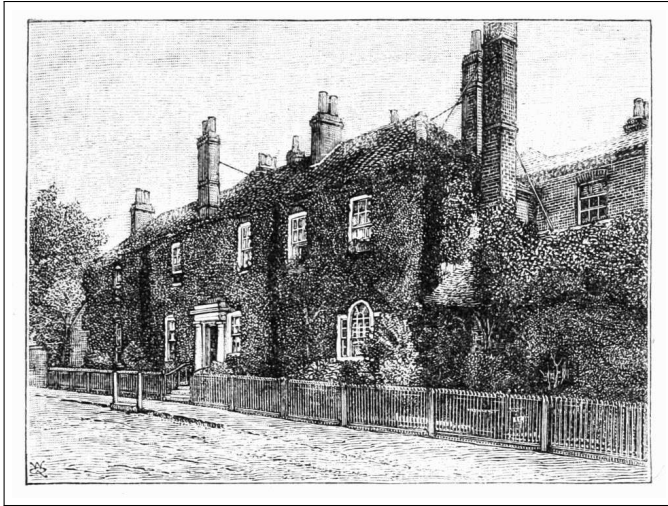
FIGURE 11.4: STREET VIEW, HERSCHEL HOUSE, SLOUGH
